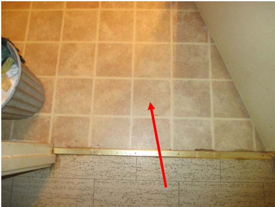
Photograph No. 2 – Unit 107 (Washroom) Asbestos-containing brown square pattern vinyl sheet flooring
