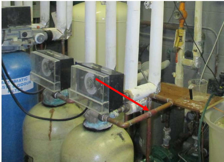
Photograph No. 3 – 1 st Floor Mechanical Room Lead solder on pipe connections
