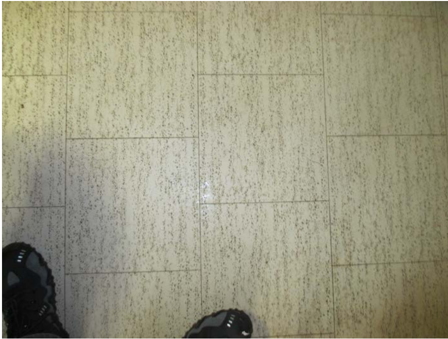
Photograph No. 1 – Unit 107 (Front Entrance) Asbestos-containing 12" x 12" white with black dots vinyl floor tile
